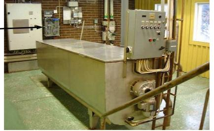
The first Siljan RotoMaster SF 17 drum thickener (above) was delivered and installed 1989 and is still in service and in excellent condition. This unit thickens sludge from a sedimentation tank and delivers the outgoing sludge to a digester. The Siljan PolySave, seen in the back-drop at the arrow, significantly enhances the performance of the Siljan RotoMaster.
